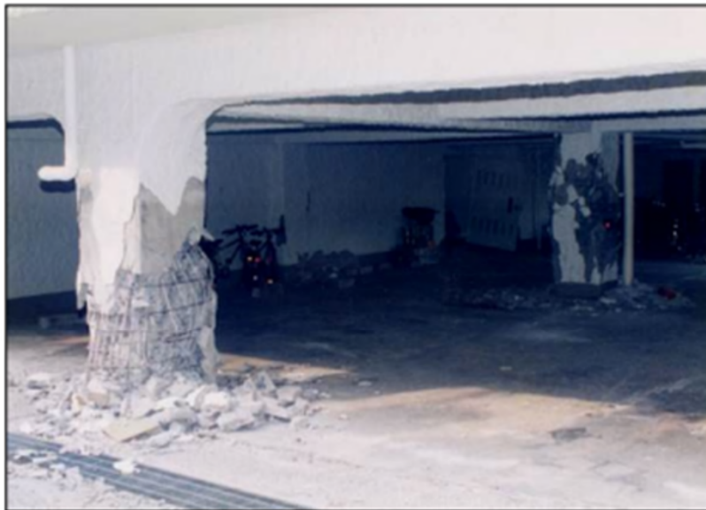
Shear Failure
